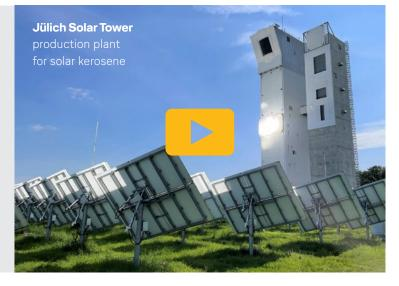
The process developed by Synhelion, which has already been verified several times on a small scale, makes it possible to remove  $CO_2$  from the atmosphere and convert it into a synthetic gas using concentrated sunlight and water. This process can then be used to generate fuel. These sun-to-liquid fuels release only as much  $CO_2$  as was previously removed from the atmosphere.
